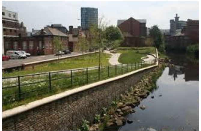
Figure 2: Dual function - park and defences at Nursery Street
