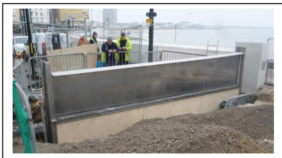
Hydraulic floodgate during installation, Margate
