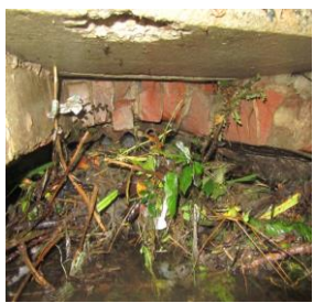
Blockage of culvert resulting in flooding, and debris removed from Culvert, Purzebrook Case Study
