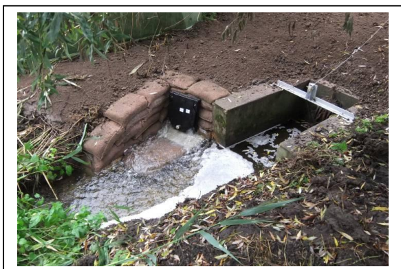
Outfall and tide flap to the land drain, next to the old tide flaps of the main streams (Pin Mill)
