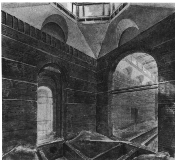
Fig. 1.1 - Dulwich Picture Gallery, drawing of a construction phase with heating pipe channels.
