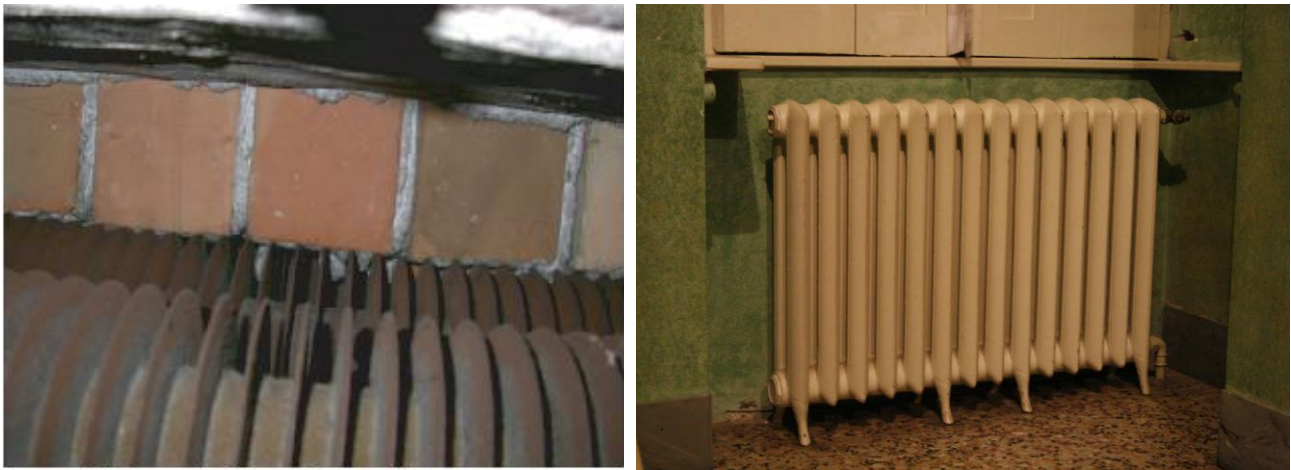
Fig. 4.7 – Finned tubes inside the ovens and a radiator in the exhibition rooms.
