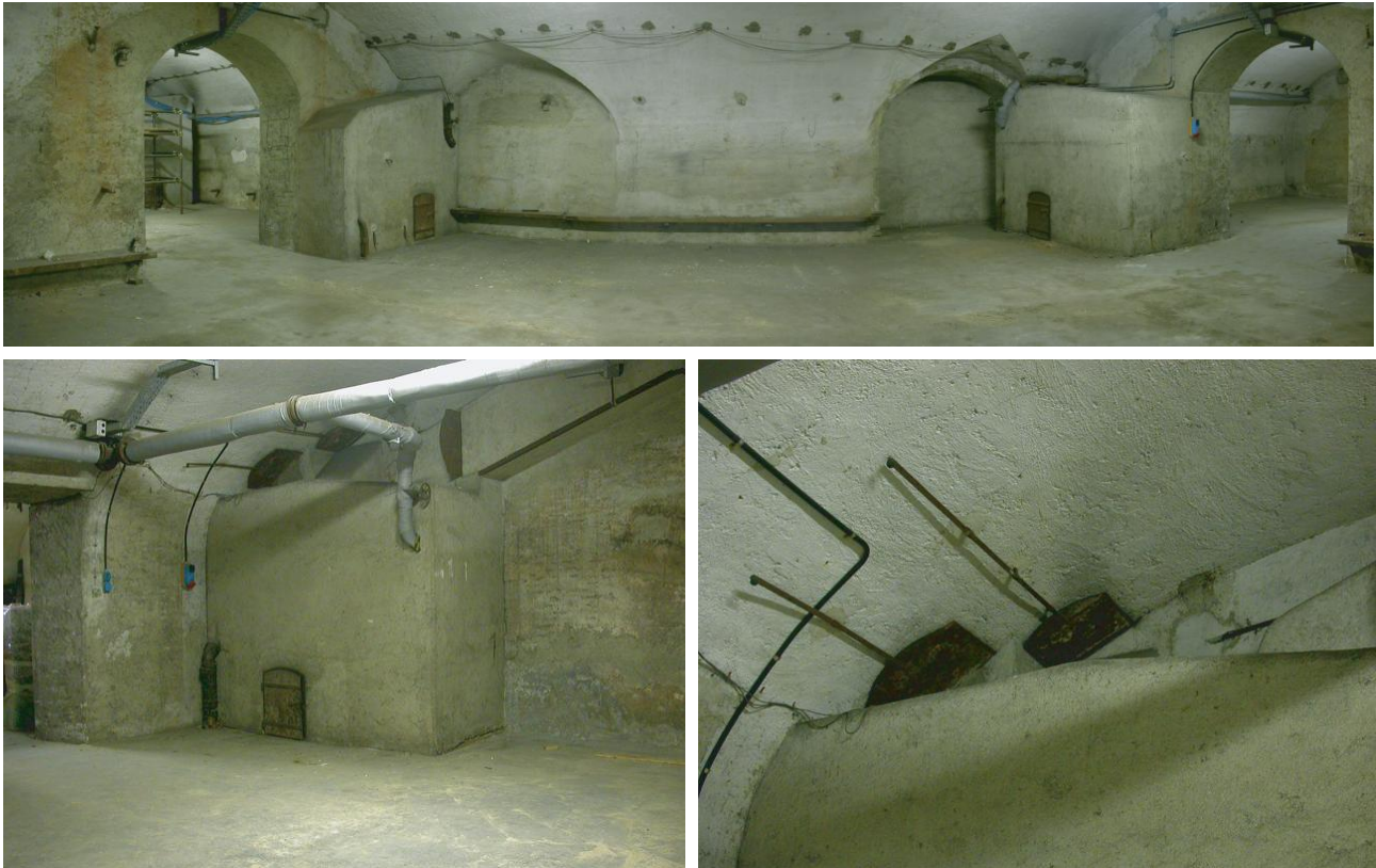
Fig. 4.6 – Meissner ovens in the underground level of the Villa before the 2002/06 interventions
