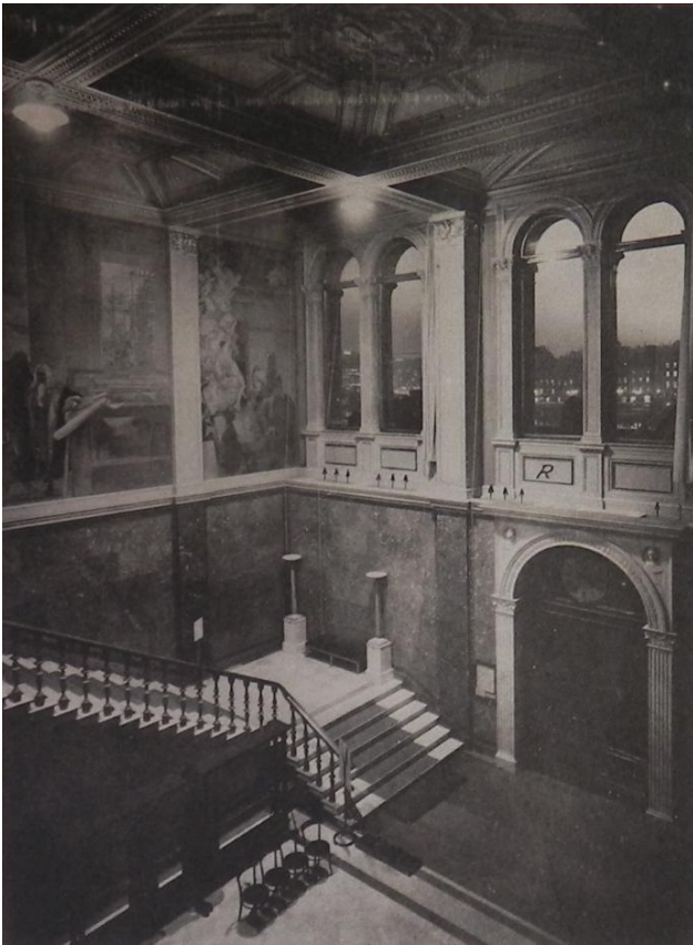
Fig. 1.15 – Nationalmuseum, Stockholm: entrance hall with air inlets (arrows) and hidden radiators (R); exhibition room with air intake and extraction.
