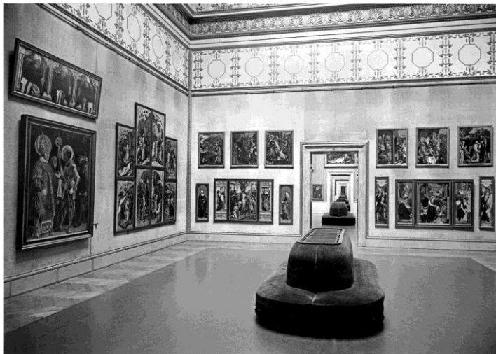
Fig. 1.4 – Alte Pinakothek, an 'enfilade' of radiators hidden by seats in a 1926 picture
