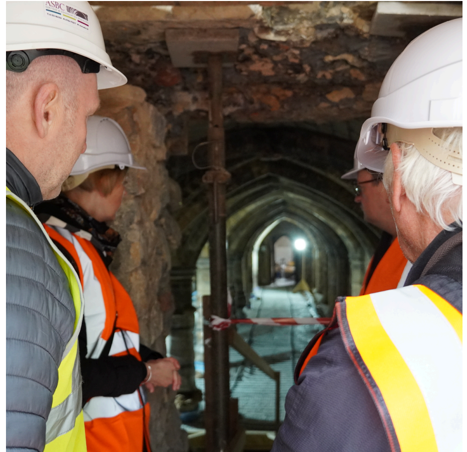
Hard hat tours at Greyfriars, Lincoln which are a typical part of heritage projects which have an activity programme and capital works.
